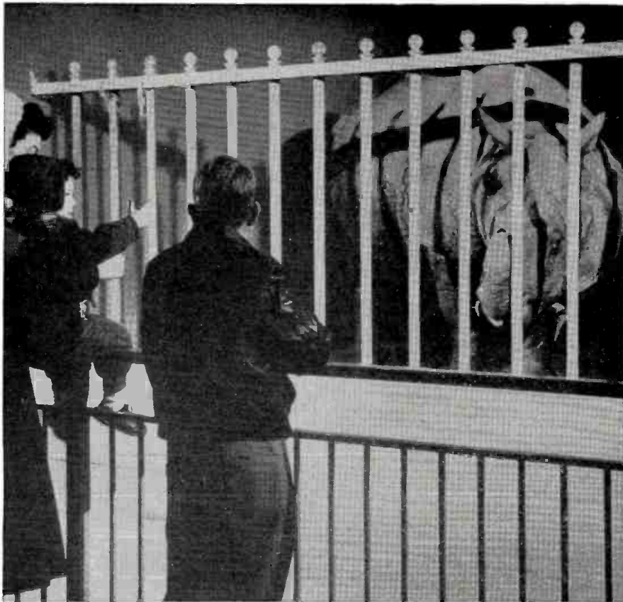
Kashi Ram is an Indian Rhinoceros at the Chicago Zoological Park, Brookfield, Ill. He's 5' 10" high, 12 feet long, and weighs 4,000 pounds. United States Steel built and erected the rhinoceros-proof fence at the front of Kashi Ram's cage. The bars are 1½" (outside diameter) extra-strong pipe welded through heavy steel channel sections.
