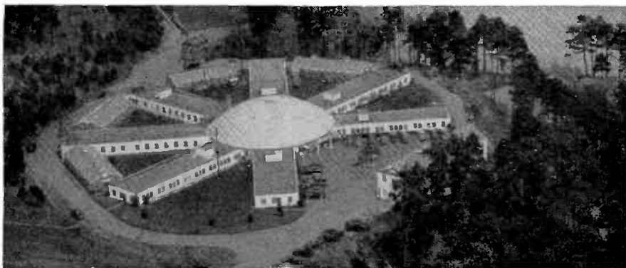
There's a Steel Hotel in Georgia. It's built like a wheel, with a 1500-seat auditorium for the hub. The wings radiate like spokes of the wheel, so that every guest has an outside room. Steel construction allows greater comfort per dollar of cost.
